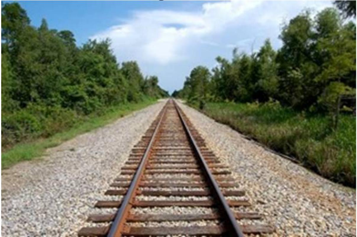
**The U.S. standard railroad gauge (distance between the rails) is 4 feet, 8.5 inches.**
